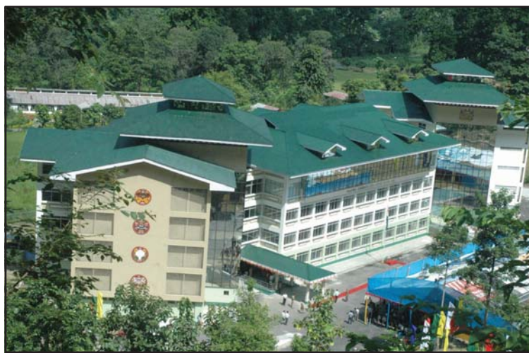
The newly inaugurated Regional Administrative Centre at Karfectar in Jorethang.
